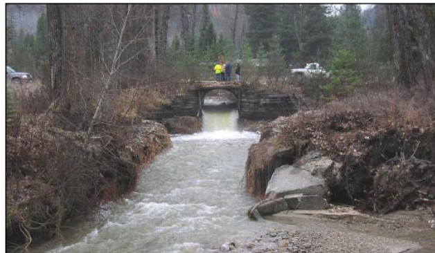
Hellroaring Creek, Idaho, culvert prior to implementation of the restoration project. The drop out of the culvert impeded fish passage into the drainage. (CFSA Appendix A)
