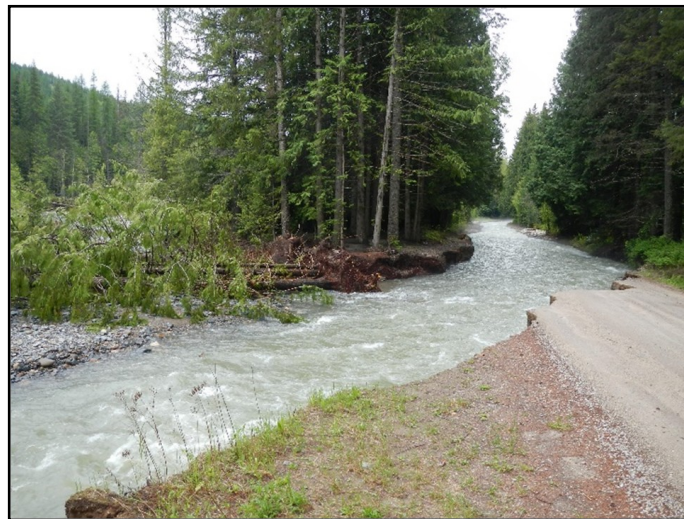
Grouse Creek Road #280 washed out on May 25, 2020.
